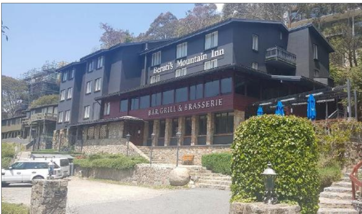
Figure 2 | View of existing building from Mowamba Place (Source: Applicant's documentation)
